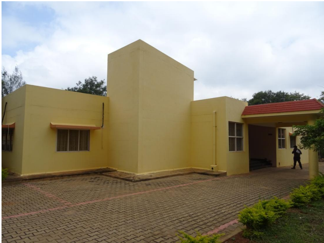
Fig 4.1: View of Guest house Building
