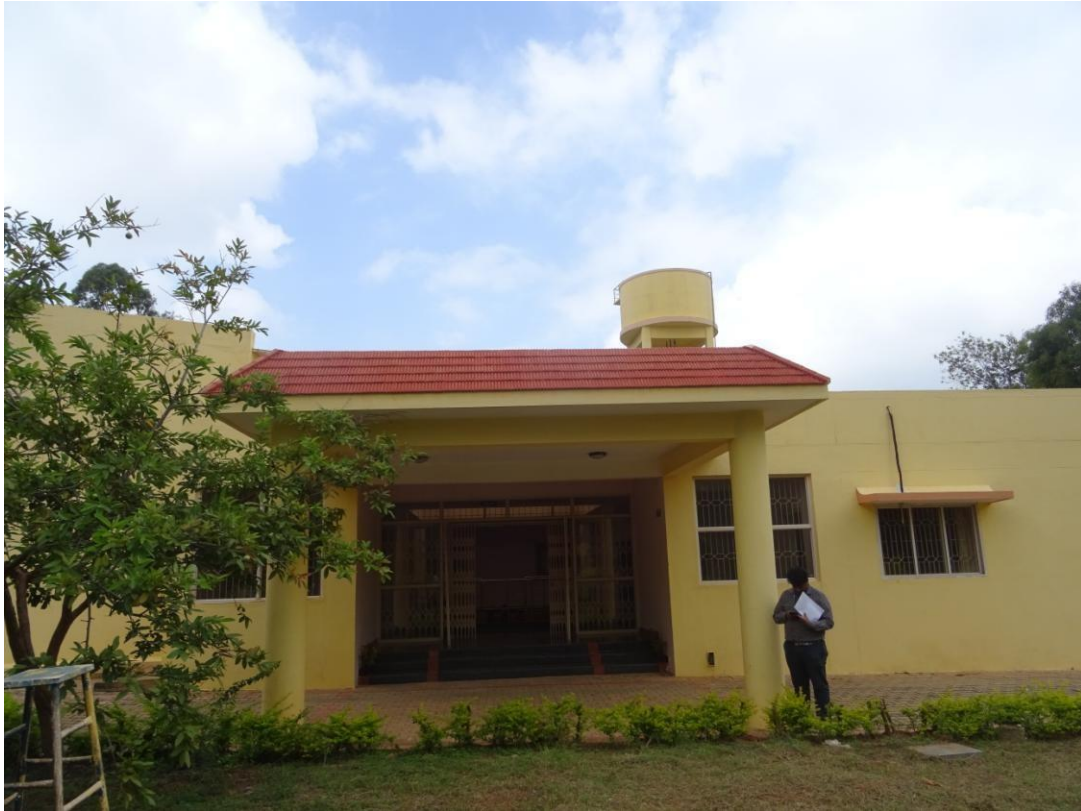
Fig 4.2: front View of guest house Building
