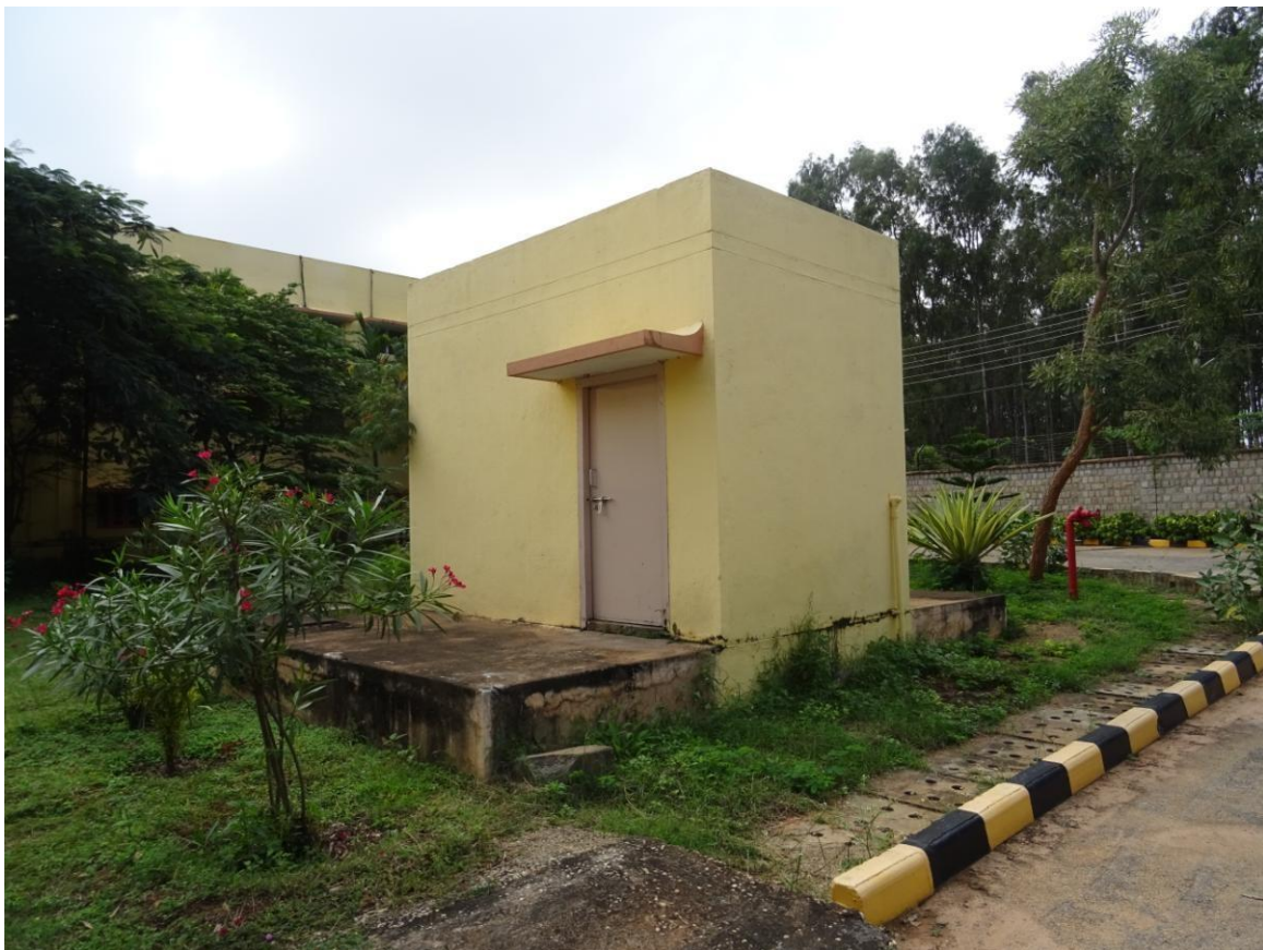
Fig 3.3: View of location of existing water storage Sump/Tank
