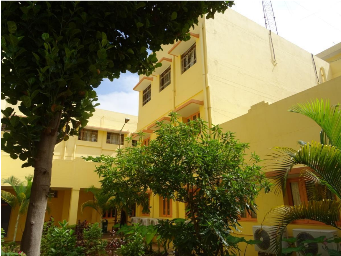
Fig 3.2: View of Canteen Building
