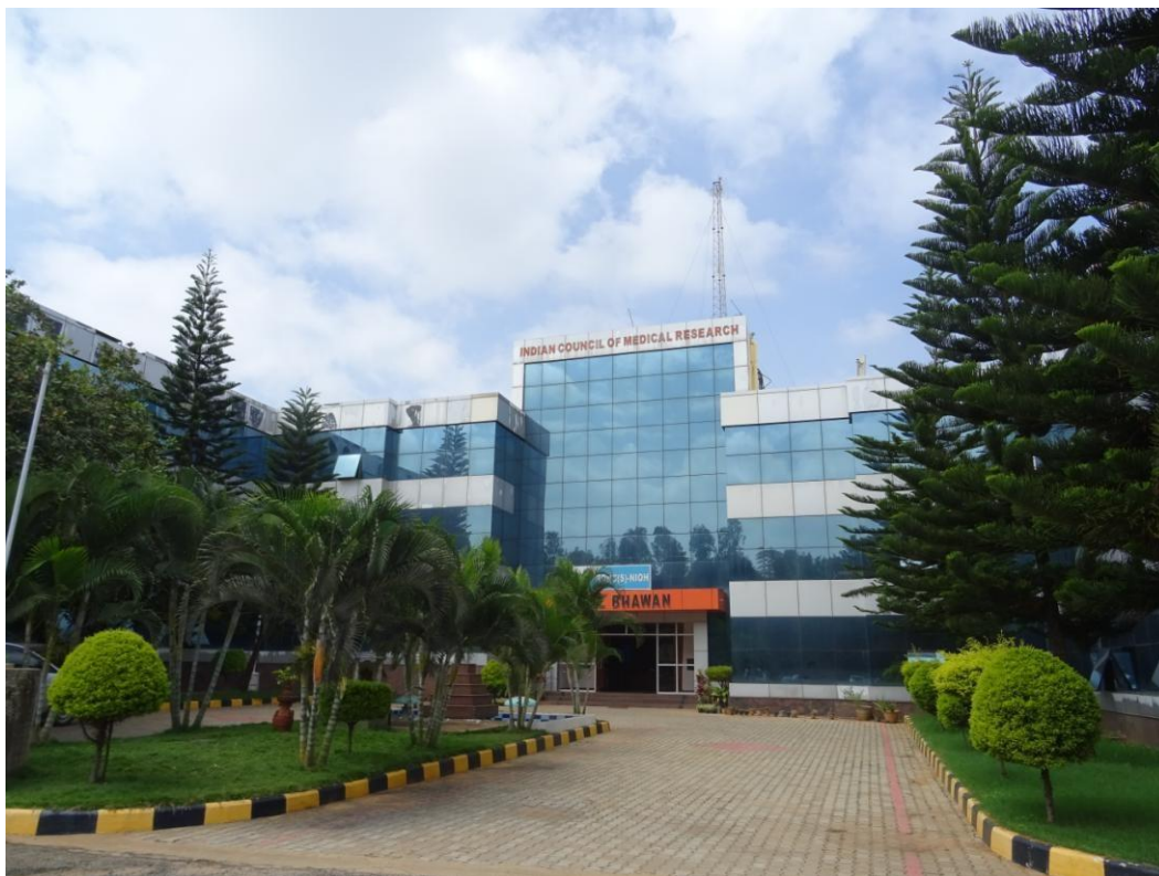
Fig 3.1: View of Nirmal Bhawan, ICMR Complex Building
